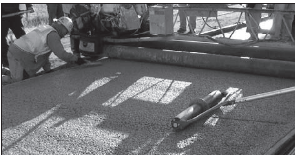
Pervious concrete placement on the MnROAD low-volume road.
